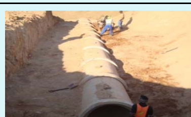
900mm Storm water crossing
