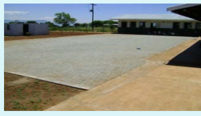
Dlangamandla brick paving complete
